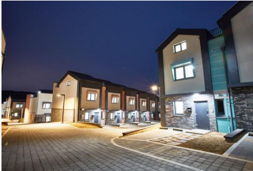
The solar-powered RoRen House complex built by a government consortium led by the Ministry of Land, Infrastructure and Transport and Korea Land & Housing Corp.
